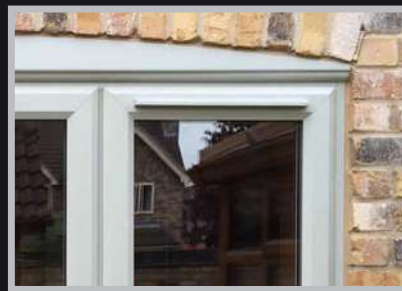
Trickle vent through a Rebated Sash
