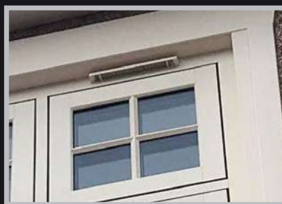
Trickle vent through the Flush Sash outer frame
