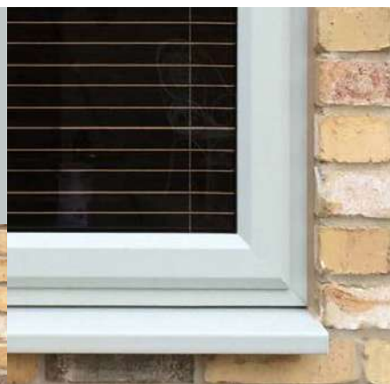
Welded joints on both outer frame and Rebated Sash
